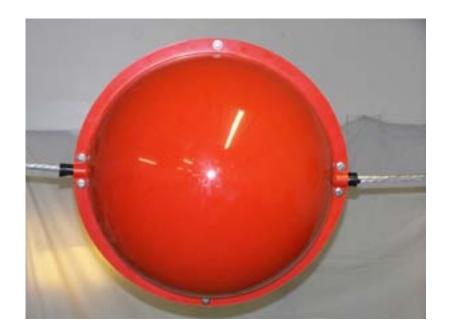
Here's one solution to the potential hazard of overhead wires in scrap yards. Our friends at Keywell have attached power line warning markers to the lines in their yards where a crane might come into contact with the wire. These markers are identical to the ones you've seen around airports and hospitals to warn aircraft of overhead power line hazards. It's an innovative way to reduce this common hazard.
