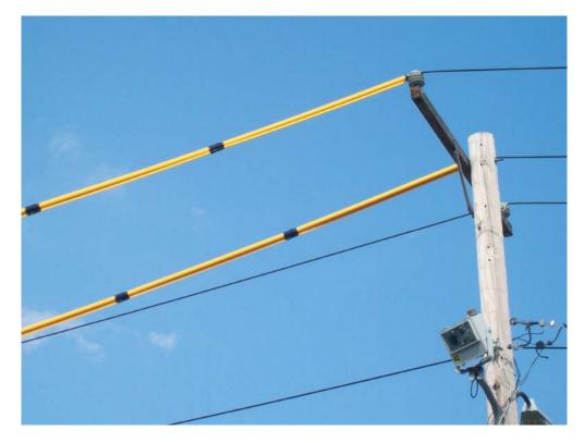
Installing power line hose in areas where mobile equipment or raised truck beds travel under electric lines is one way to reduce the risk of electrocution and property damage. Contact your local industrial electric contractor for information about installing these in your operation.
